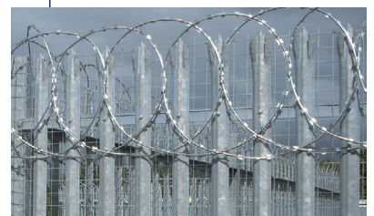
At the upper part of palisade fencing
