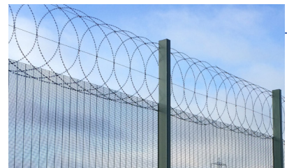
At the top of 358 high security fence
