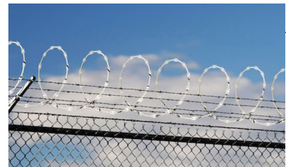
For road restricted area protection
