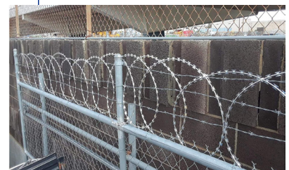
At the top of fence gate
